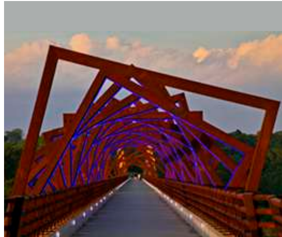
HIGH TRESTLE, CENTRAL IOWA
